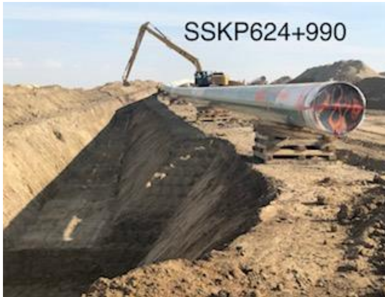
Crews using excavators to create sand bed before lowering
