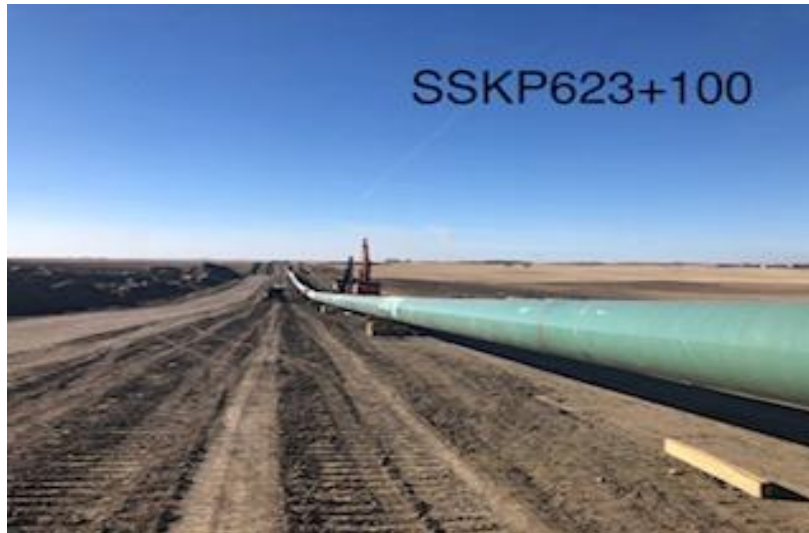
Beginning of the ditch process
