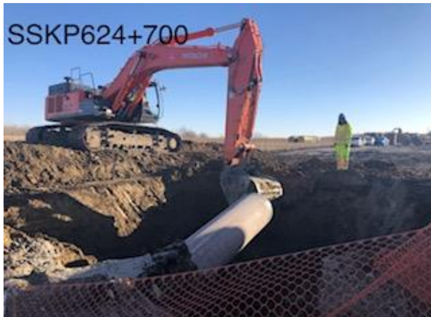
Excavating around pipe in preparation for hydro test
