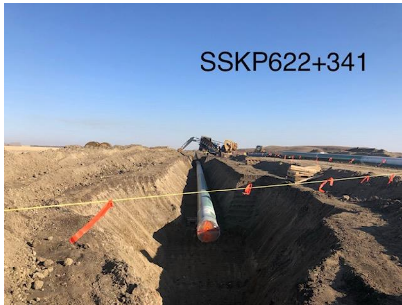
Lowered in mainline section
