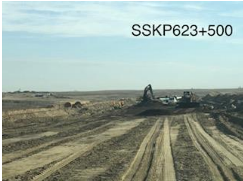
Backfill process on west of Chapleau Lake
