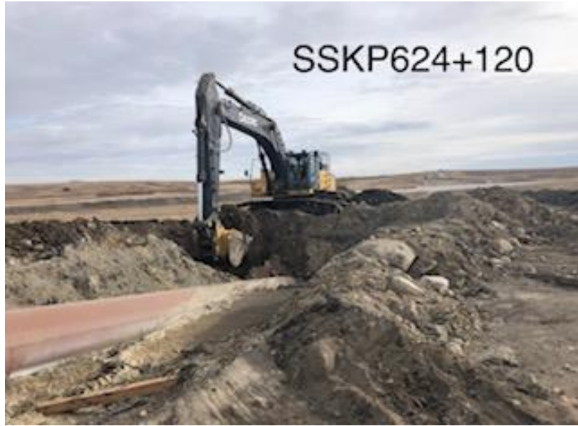
Excavating around HDD area for cut out
